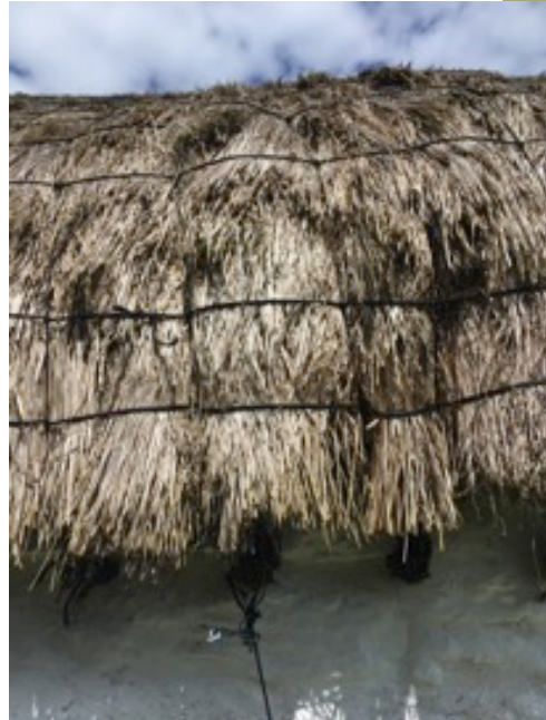
Above: Rye thatch on barn and museum roofs Below: Abandoned barn and new corrugated iron roof
